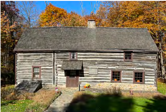
The Shelter House - 1743
