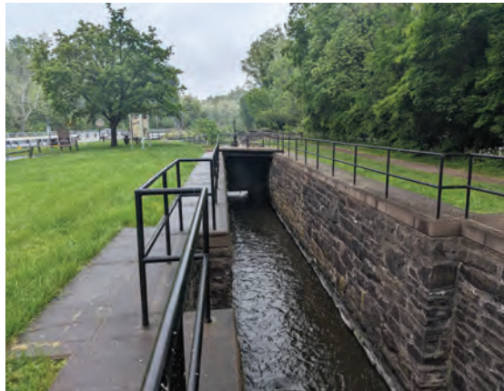
Delaware Canal Lock 21
