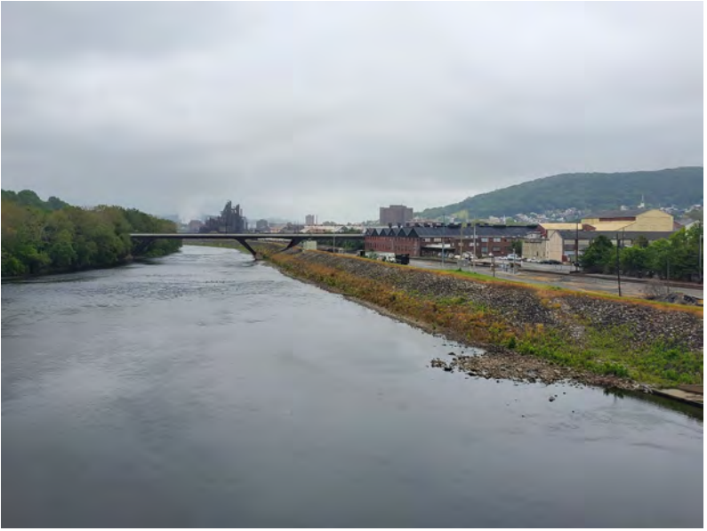
View from Hill to Hill Bridge looking east, 2023
